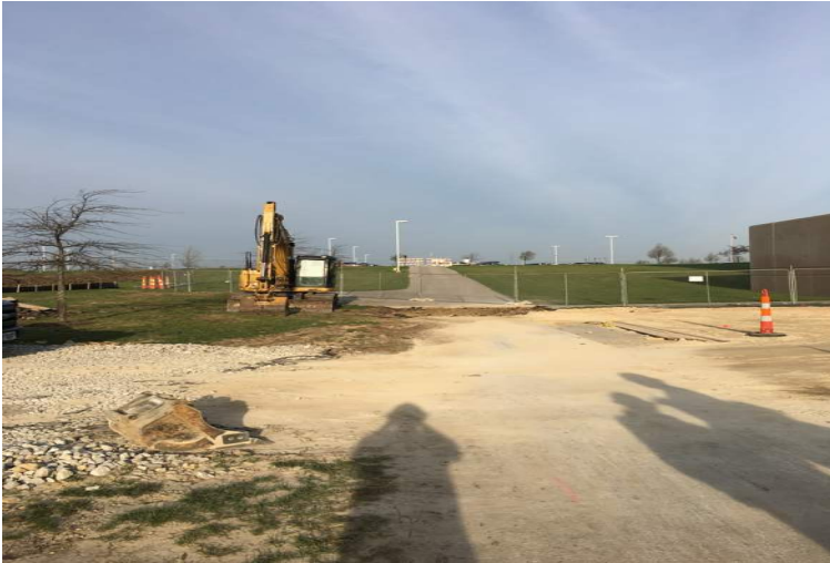
Storm Boxes Being Excavated
