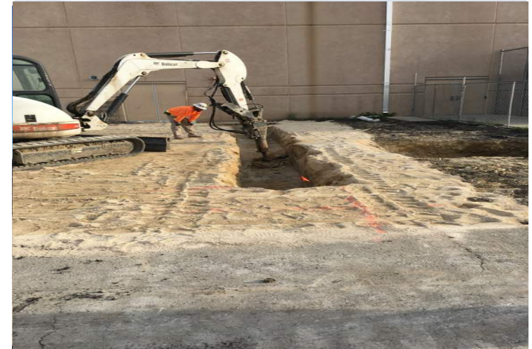
Chipping Rock in Bottom of Footings
