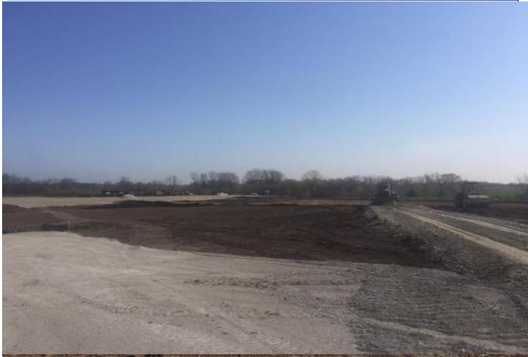
Access Road Installed to Bldg Pad
