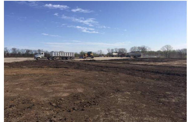
Bldg Pad - 100% Complete
