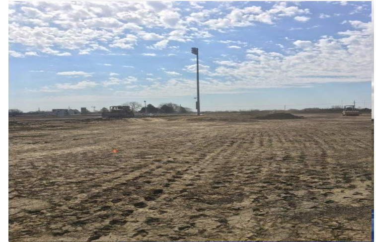
Grandstand Building Pad
