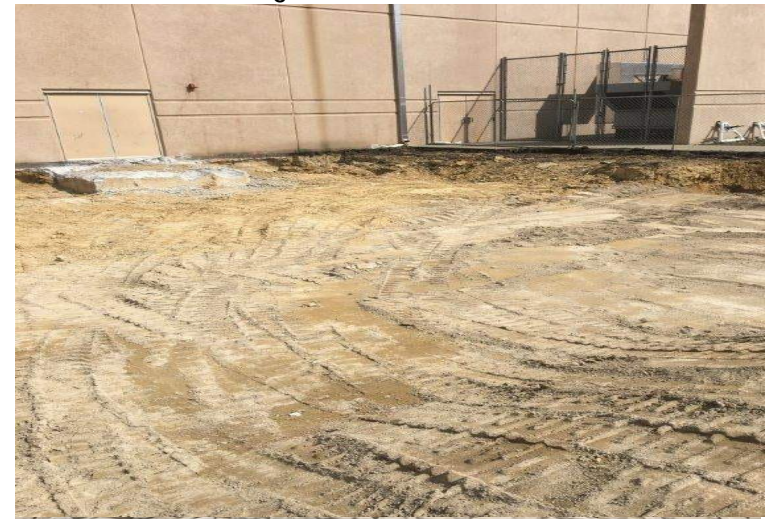
Building Addition - Mass Excavation
