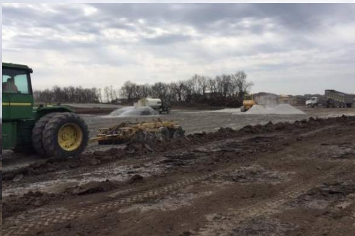
Building Pad Installation
