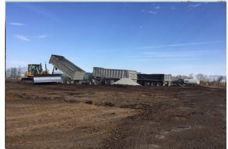
Construction Road Installation
