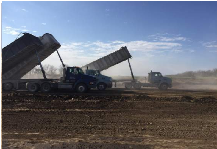
Building Pad Installation
