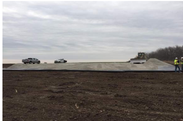
Building Pad Installation
