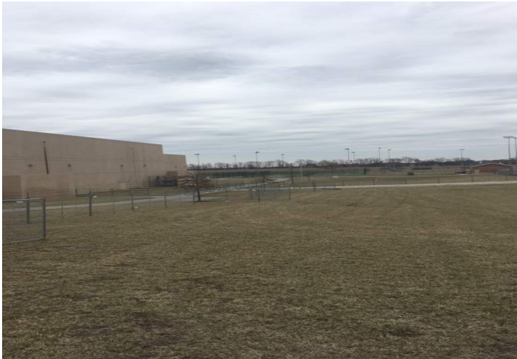
Construction Fence Install
