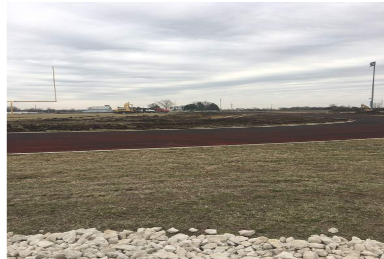
Football Field Clearing
