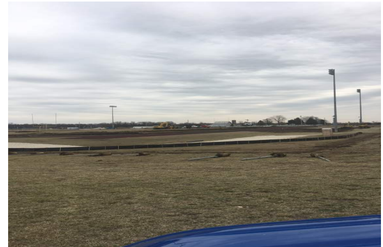
Football Field Clearing
